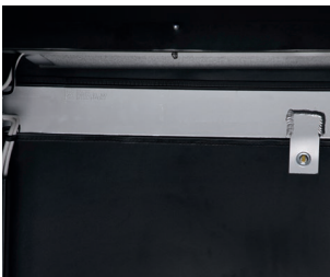
Optimised Cooling System for High Ambient Temperature
